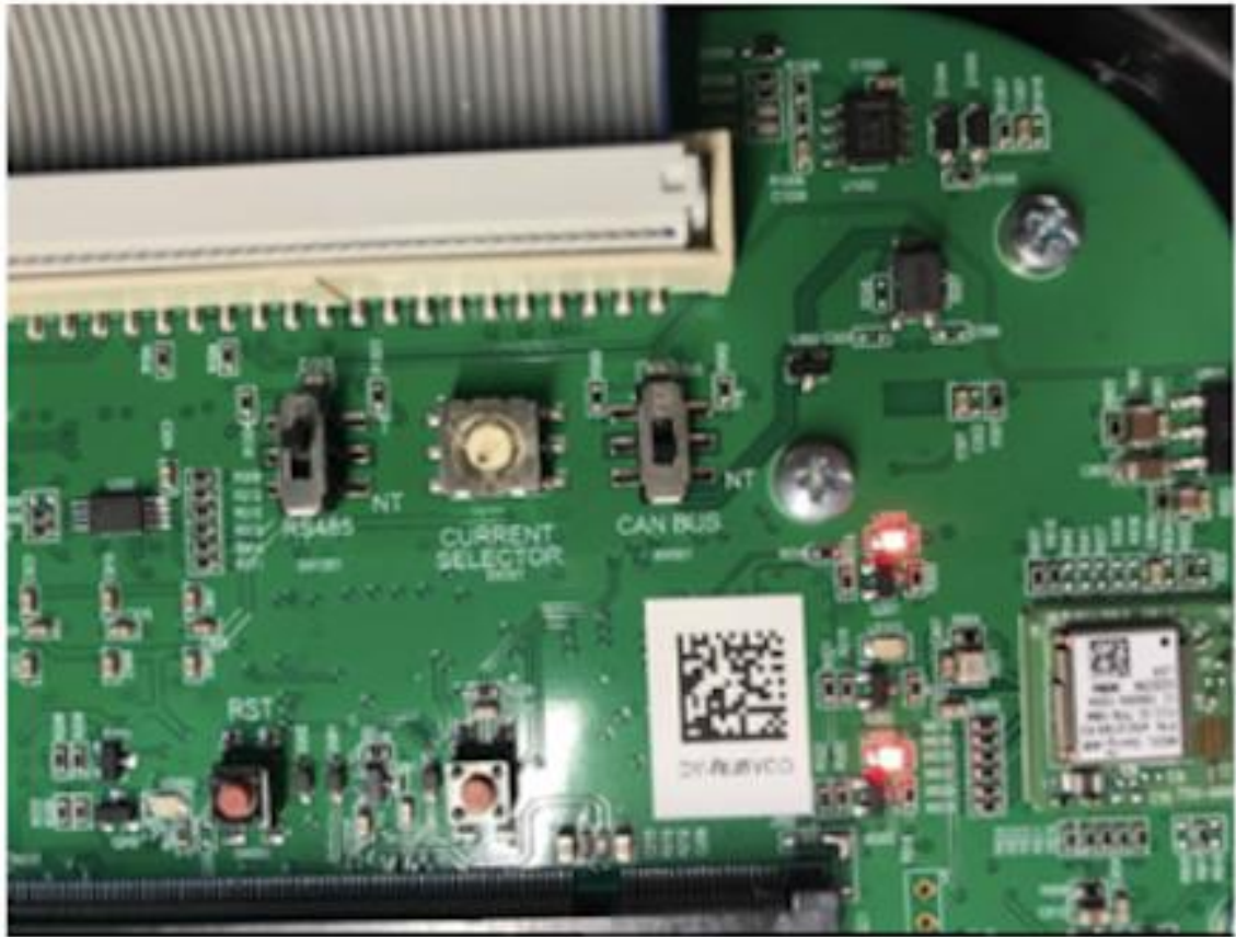
Close up RS485/ CAN bus switches
